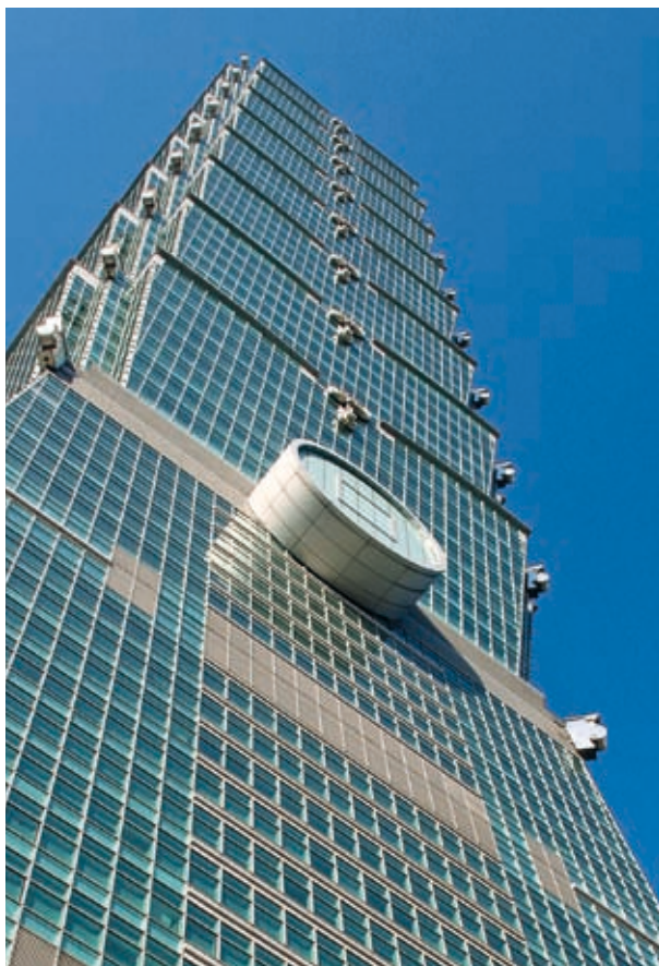
5.000 m of façade sealing at Tower 101, Taiwan.
