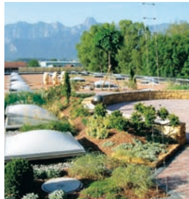
Left picture: Roof sealing sheets at Makino Engine works, Japan.
