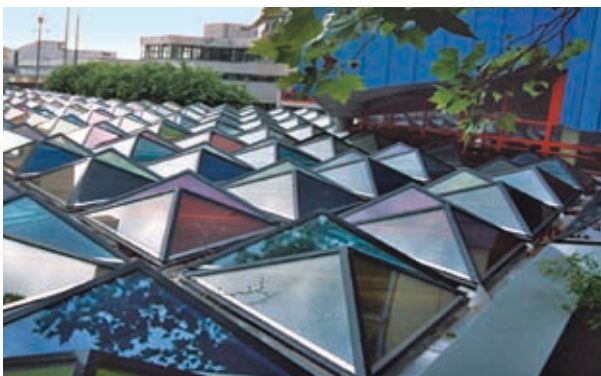
Gutter coating at the landmarked pyramidal glass roof, University of Constance, Germany.
