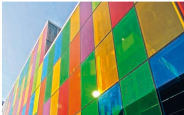
Façade sealing at Convention Center Montreal, Canada.
