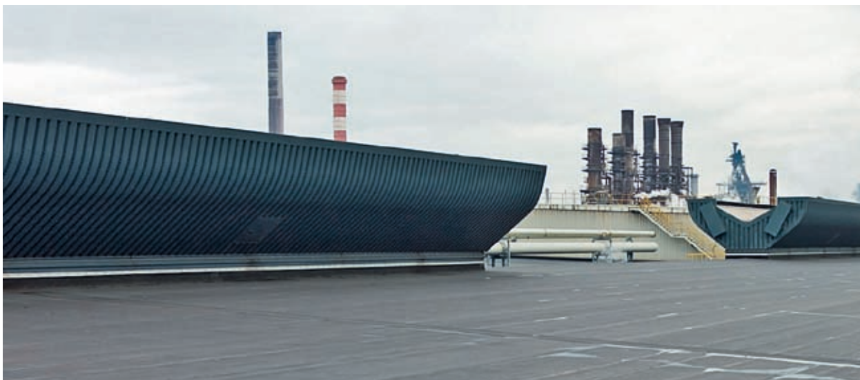
EPDM sealing at steelworks Dillinger Hütte, Germany.
