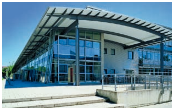
Façade sealing at the Technical University Rosenheim, Germany.
