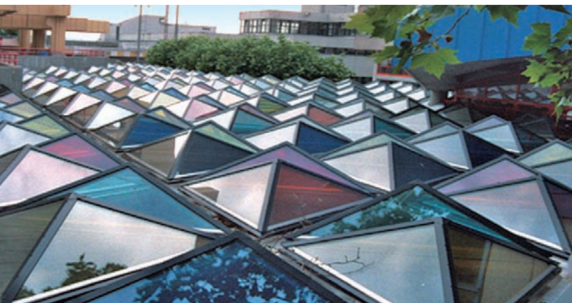
Gutter lining at the heritage-protected pyramid roof, University of Konstanz, Germany.
