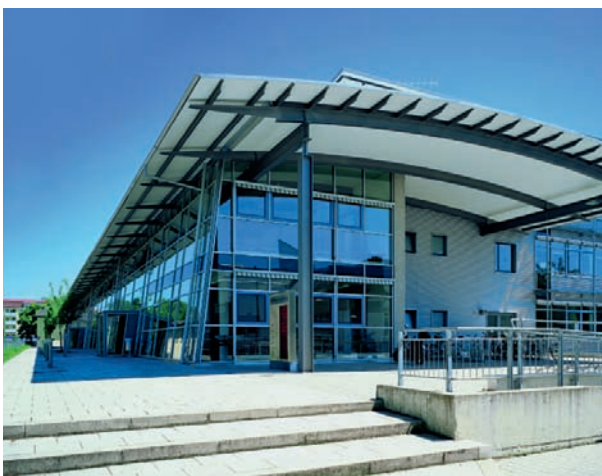
Façade sealing at university of applied sciences, Rosenheim, Germany.
